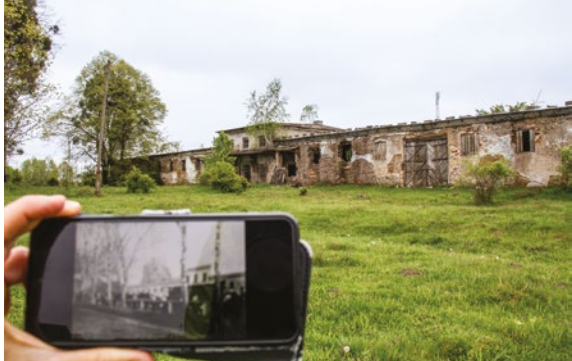
Fig. 7 Field survey in Hruszów, ruins of the barracks buildings juxtaposed with an archival photo. Source: photo by E. Józefowicz.
